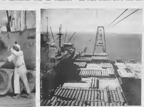
View of a freighter berthed at the artificial sea-level three miles off the mainland of Ras el Mish'ah, Saudi Arabia. The Skyhook machine rode on cables slung from a parade of 90-foot high A-frames.
